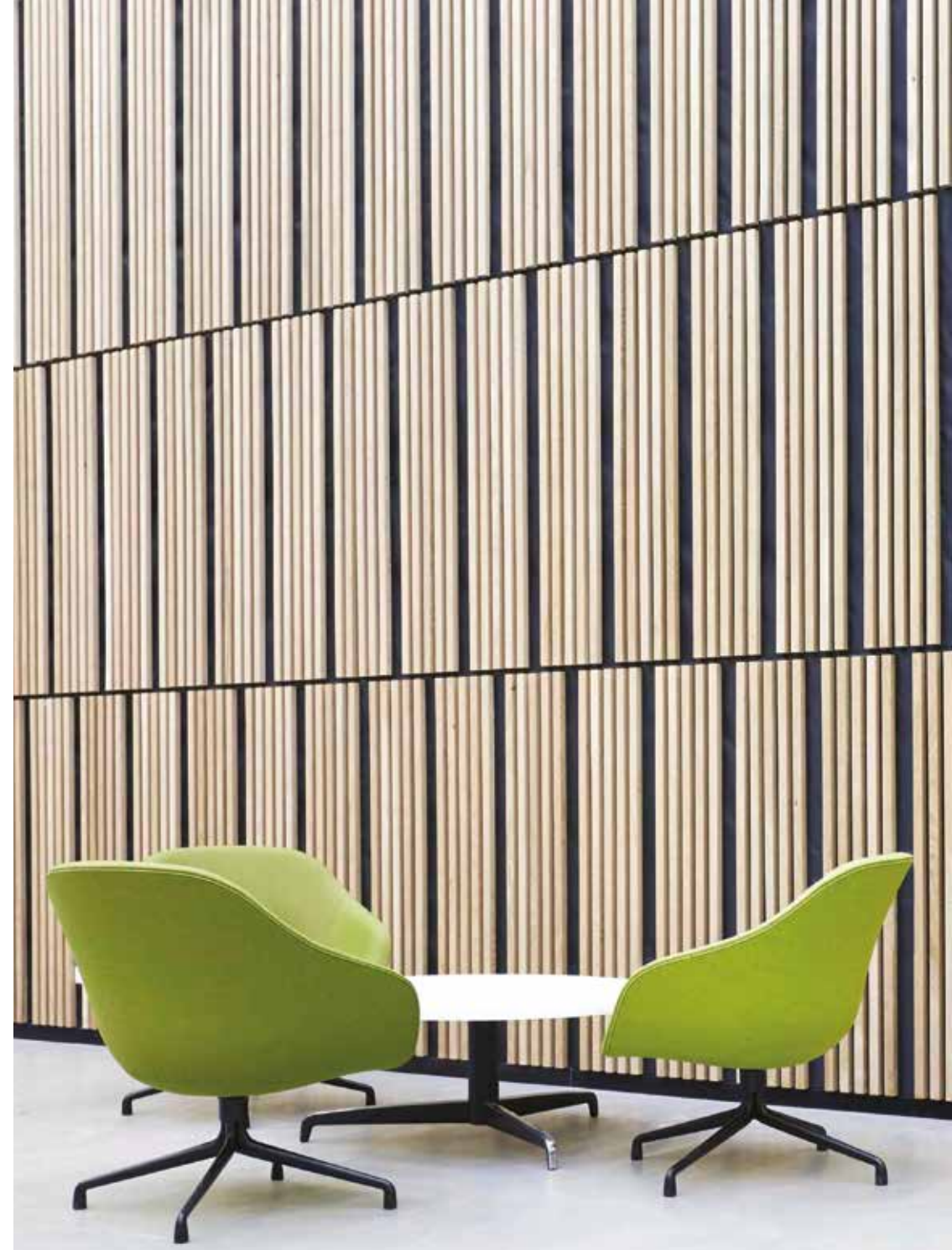
Interior sound-absorbing construction, treated with C260.
